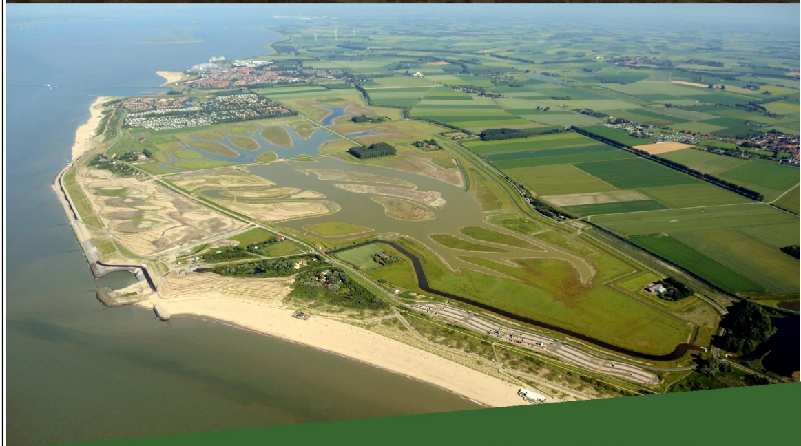
Waterdunen tidal lock and state of works
